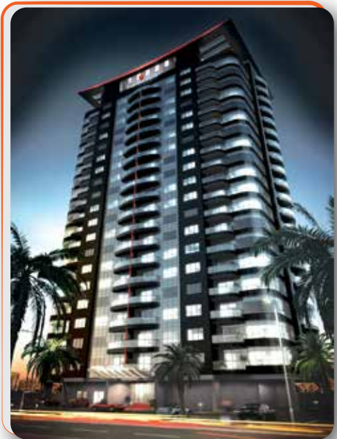
LAMBORGHINI RESIDENCE TOWER IN DUBAI SPORTS CITY
